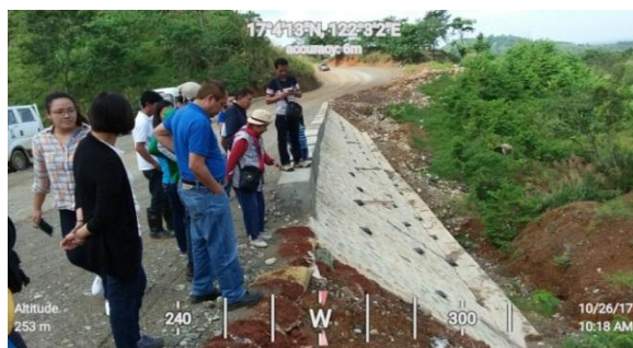
ENR Officer together with the committee inspecting one of the structures along the road during the RMFPC visit to the IDRRIP
