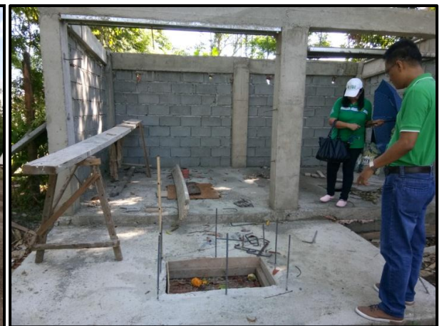
Cabagan District Hospital New Infectious vault under construction
