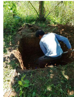
Establishment of chemical waste disposal pit.
