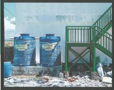
The Installation of Rain Barrels. The CCSTHS installed rain barrels to different designated areas around the school (beside Admin building, right side of the gymnasium and left side of AFA building). These barrels are use to collect and store water from roofs for future use such as watering gardens and cleaning.
