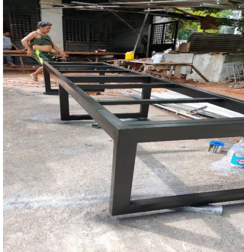
Fabrication of plat form
