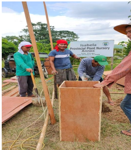
construction of Animal shelter
