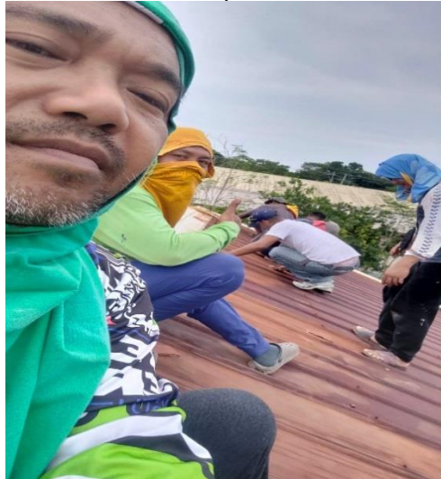
construction of x-ray room at Manuel A. Roxas District Hospital
