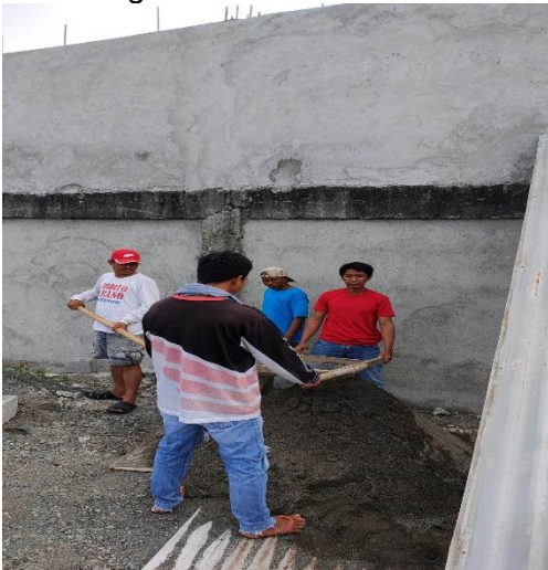
Plastering of wall
