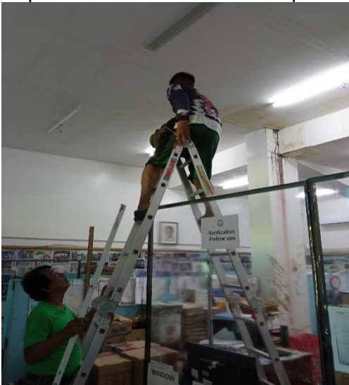
Replacement of fluorescent lamp
