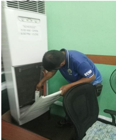
Cleaning of Air-conditioner
