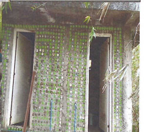
Constructed compost room
