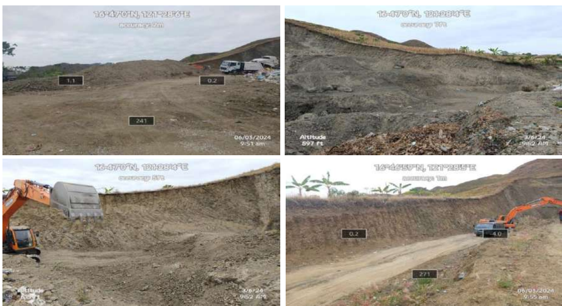
Area 2: Excavation of Cell 2 of the Sanitary Land Fill.
