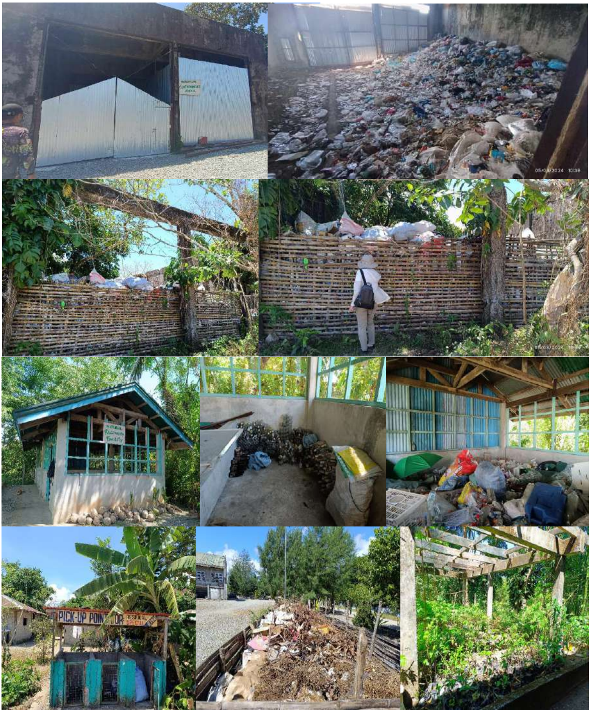
Maconacon, Isabela Disposal Facility at Brgy. Malasin, Maconacon, Isabela
