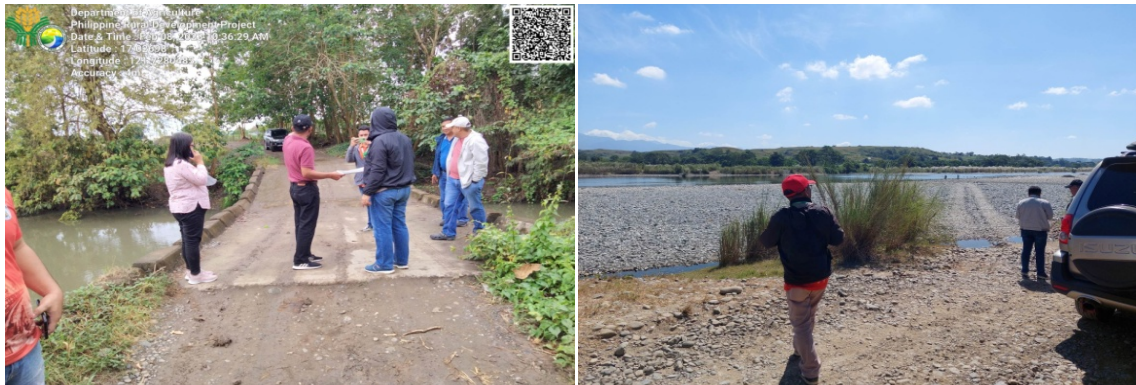
Rehabilitation of Bridge
