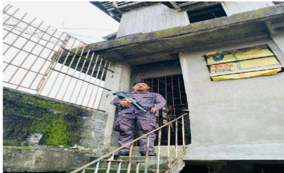
Fig. 8- Photograph showing the Tower 1 Guard house of Isabela Provincial Jail
