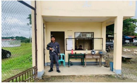
Fig. 7- Photograph showing the Gate Guard house of Isabela Provincial Jail.
