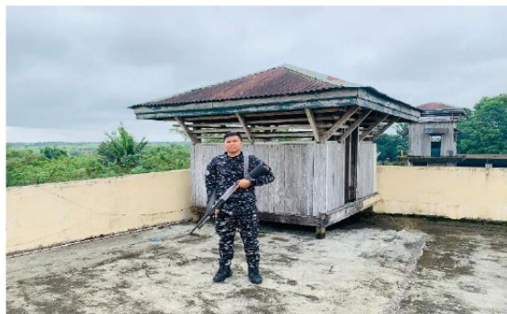
Fig. 9- Photograph showing the Tower 2 Guard house of Isabela Provincial Jail
