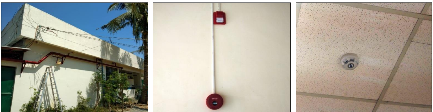
Smoke Detector and Fire Alarm System
