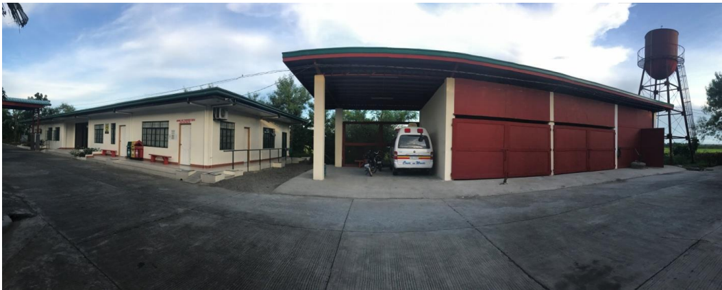
Newly constructed Motor Pool
