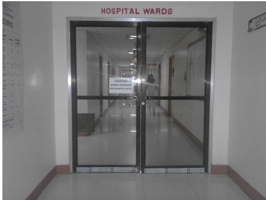
Newly replaced ER glass doors (to Wards)
