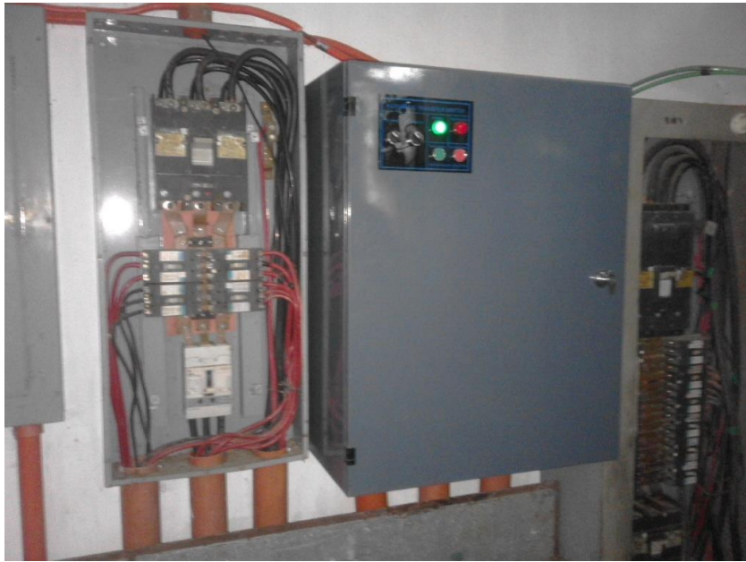
Newly installed Automatic Transformer Switch acquired through PLGU
